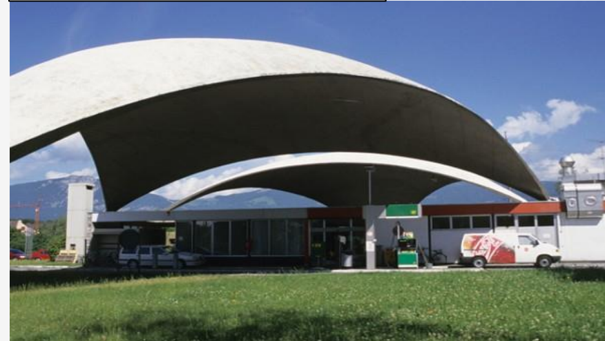
Photo - Station-service de Deitingen
