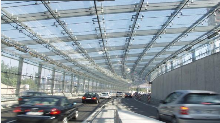
Photo – Tunnel antibruit - Munich
